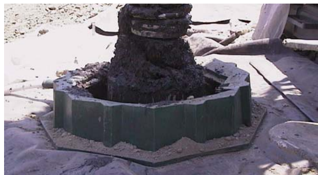
Figure 5 – Drilling in Saturated Refuse
