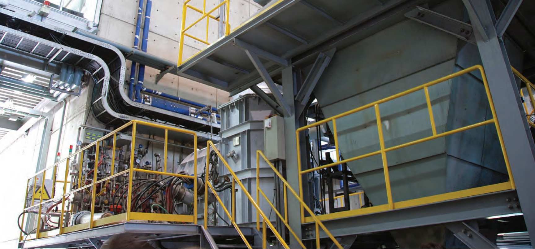
The newly started 10 ton per day GS Platch MSW conversion plant in South Korea. It uses plasma gasification to produce syngas for electrical production. Photo courtesy of David Ross, SCS Engineers.
