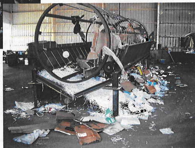
Converting to single stream: initially, the team at Escambia County looked at a star screen to provide automated OCC separation on the front end, but the benefit/cost of the system was not favourable. Instead, the County decided to fabricate a mobile trommel, which would involve some manual labour, for removal of OCC from the waste stream.
