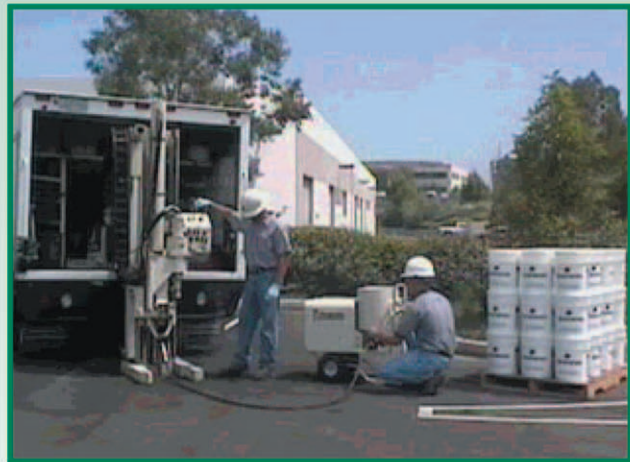
On-site direct injection of ORC
